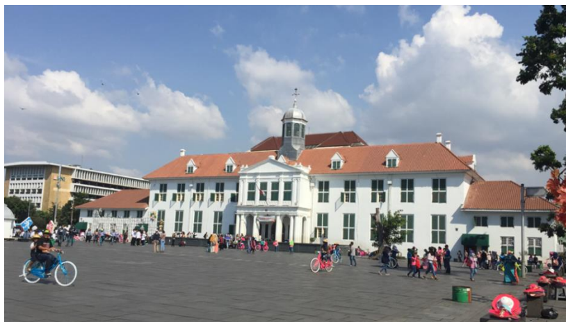
Fig. 1. The Museum Fatahillah under renovation (Purwantiasning, 2015).
