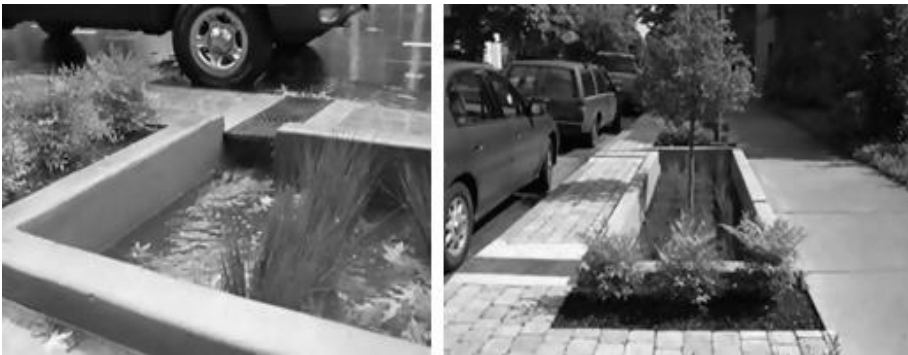
Fig. 3 Proposed drainage system on SW 12th Avenue Green Street, Portland, Oregon ( Portland Bureau of Environmental Services, 2016 ).
