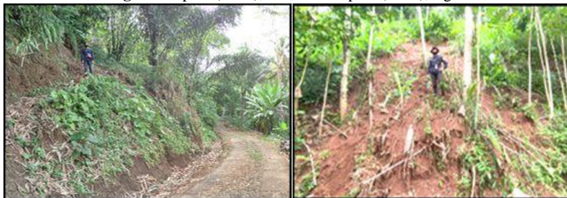
Fig. 7. Slope 3 (LR 3), left, and Slope 4 (LR 4), right.
