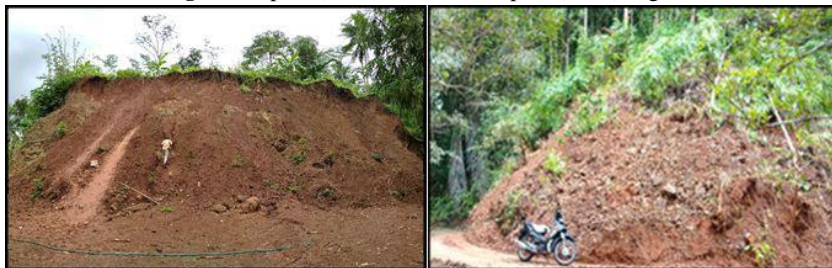
Fig. 8. Slope 5 (LR 5), left, and Slope 6 (LR 6), right.
